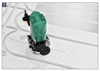
Rout a 5mm groove from the thermostat location to the sensor position and cut a 50mm square section, 5mm deep into the insulation.
