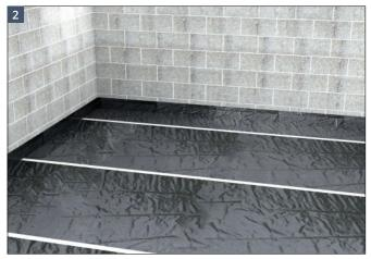
If a damp proof membrane has not already been installed within the subfloor construction, lay a damp proof membrane over the subfloor to prevent water ingress.
