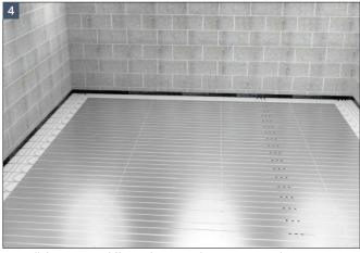
· Install the Warmup diffuser plates into the Contura panels.
