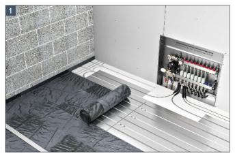
Lay a vapour control layer over the Contura system first to prevent moisture ingress.
